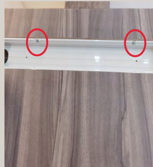
4 Fixed on the mounting plate onto the surface by drilling the screws into the screw holes
