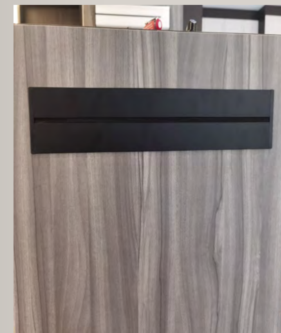
7 Installation is finished once the recessed e-Bar is fitted nicely on the mounting plate within the cutout hole
