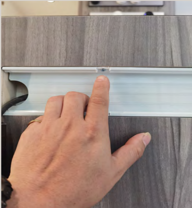
3 Identify the screw holes of the mounting plate and make sure they are aligned to the surface properly
