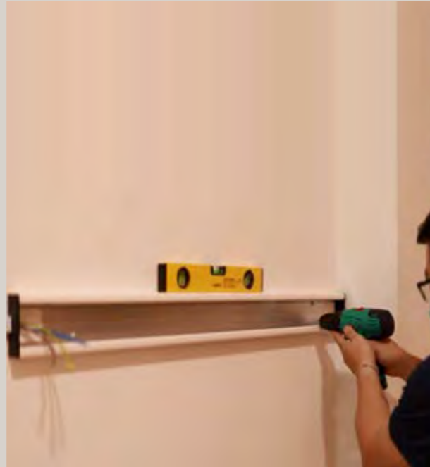
10 Secure the right side of the Power Track Housing with Wall Screws
