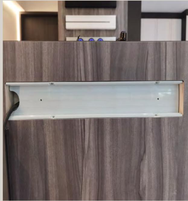
2 Insert the mounting plate into the cut out hole, making sure the "Live, Earth and Neutral" wires are inserted into the curved portion of the plate.
